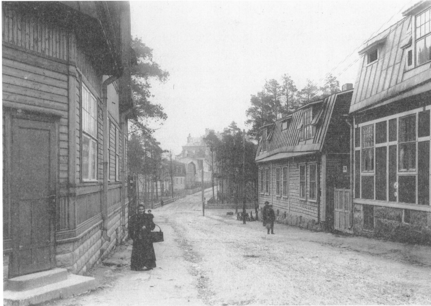
FIG. 2. The Vallila working-class housing district, Helsinki, in the early twentieth century. Solid log walls were used even in an urban context (Helsinki City Museum Picture Archives).
