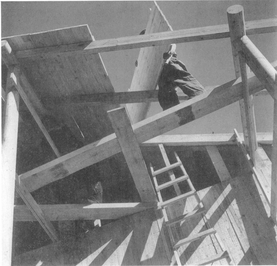
FIG. 5. Erecting an AA-system house (Museum of Finnish Architecture Picture Archives, Helsinki).
